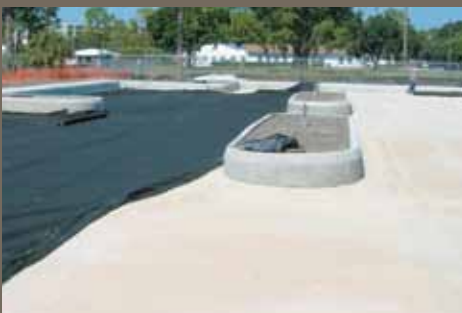
North Parking Lot geo-textile fabric layer
