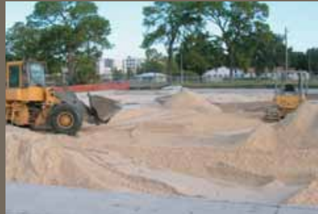
North Parking Lot fine aggregate layer
