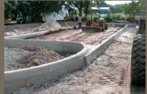
South Parking ribbon curb and 6" vertical curb
