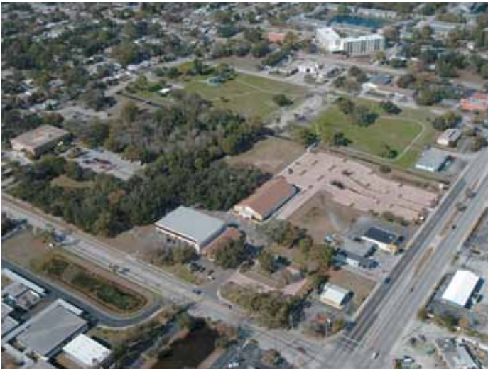
Aerial of entire site, City Hall, North and South parking lots and Towne Square Park
