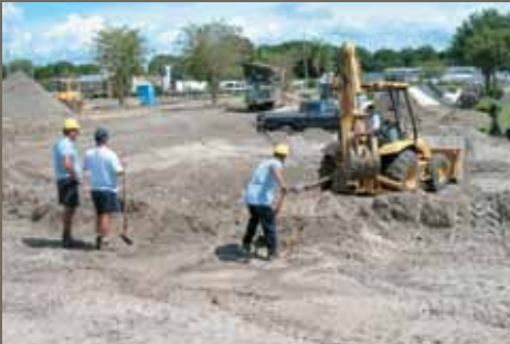
North Parking Lot Public Works Employees installing irrigation and lighting conduits
