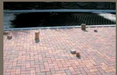
South Parking GEO-WEB and pavers
